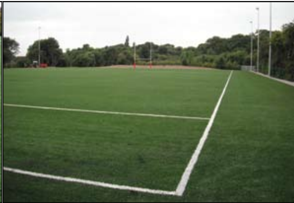
Installation at Burnage RFC.
